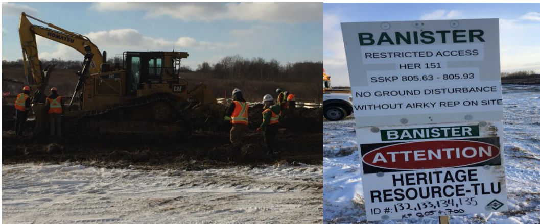
Pipestone Creek East side track hoe stripping topsoil – Archeologists and teams walking the area.
