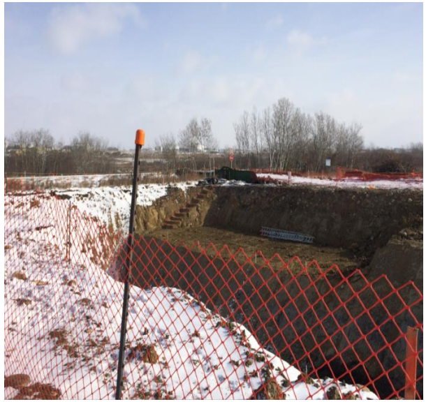
Pipestone Creek West side 805 + 700 – Track bore excavation
