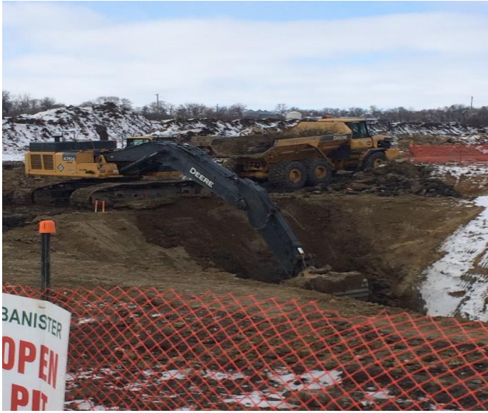
Pipestone Creek West side 805 + 700 – Track bore excavation
