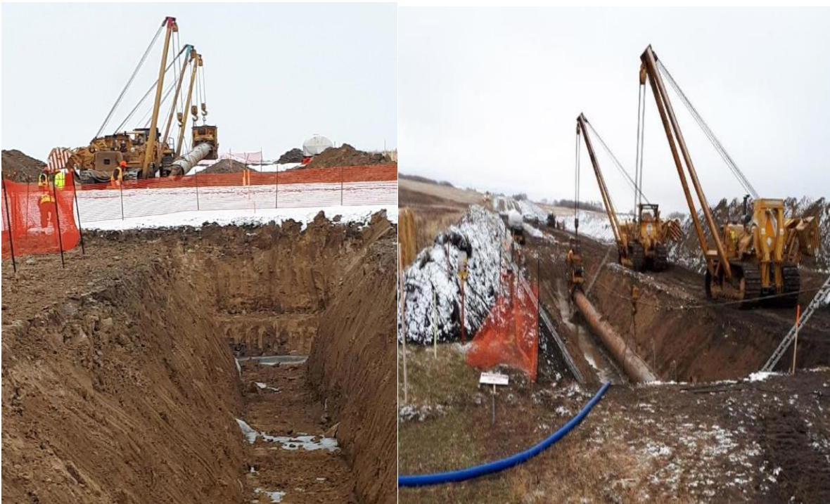
Picture left Tail ditch – Picture right bore hole entry (Side Booms)
