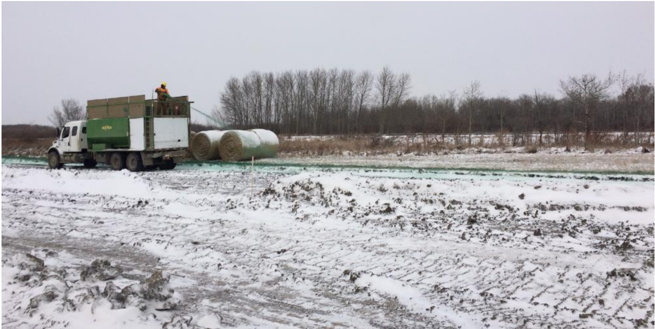
Tackifying (Soil Stabilization)
