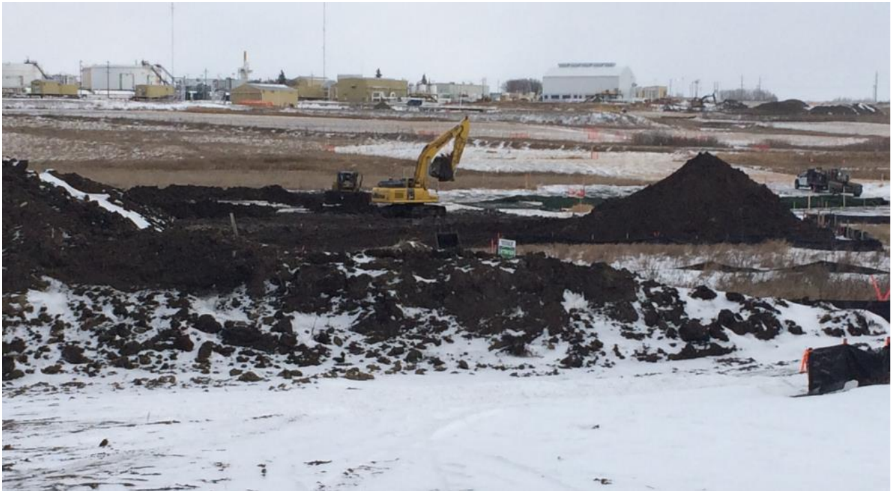
East side Pipestone Creek stripping topsoil
